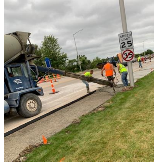
Village of Little Chute crew working on replacing the sidewalk on the Highway “N” (Community Bridge).
